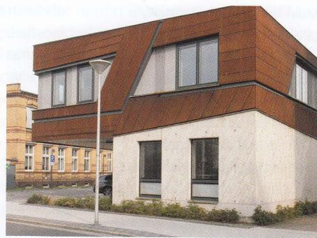
When facades are designed, for example, with weathering steel on the upper storeys and with a base in exposed concrete, corrosion and weather-related residues can discolour the concrete surface over time. PSS Inter-service offers a RAL-certified, prophylactic surface protection. PSS 20 is a thin, invisible and
